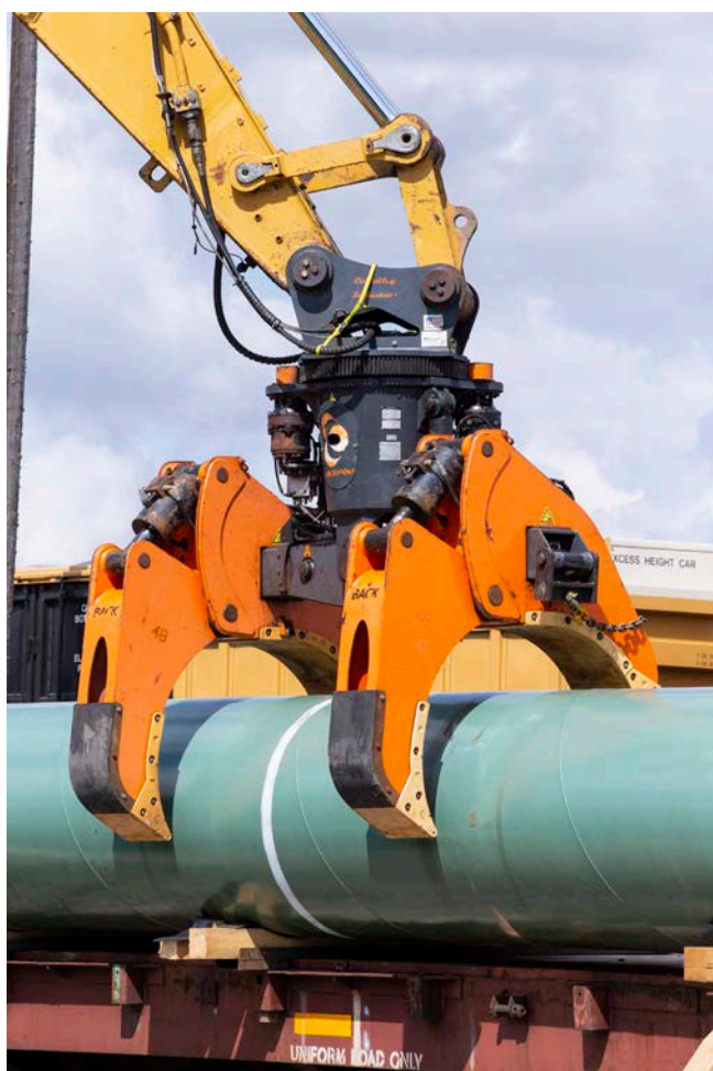
Figure 3. Wear pads protect coated pipe.
